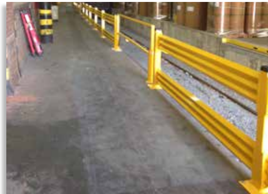
Protecting rail dock
